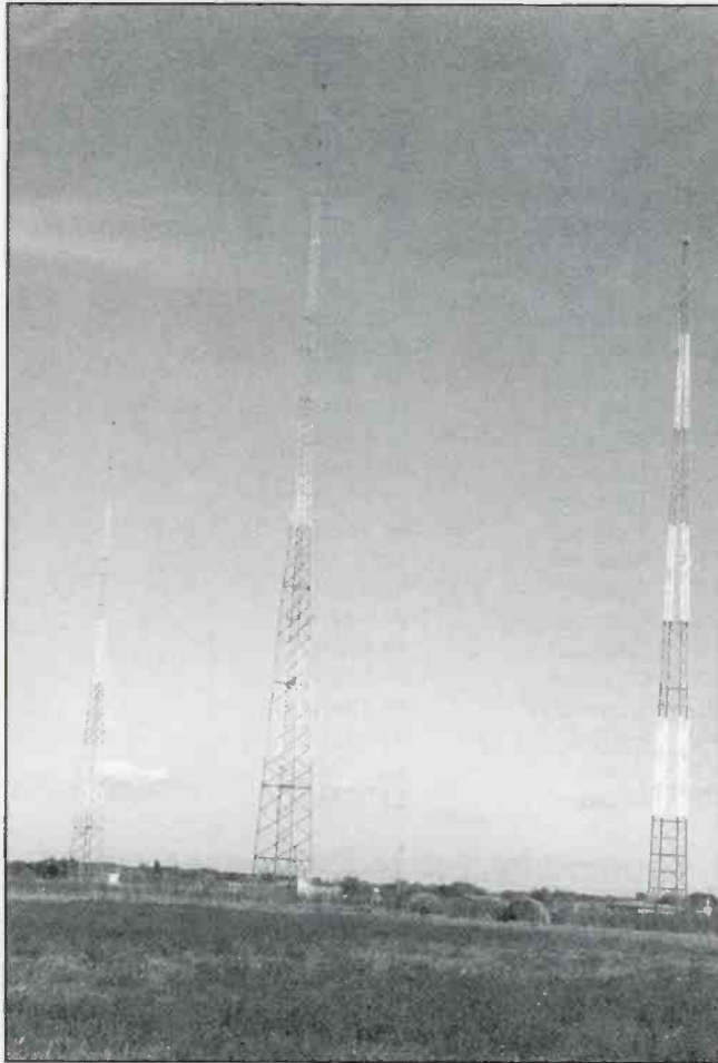
The WNFL 1360 kHz three-tower directional array. (Photo by U.R. Albrecht)
